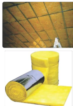
Figure 31.3 Fibreglass is used for insulating walls and ceiling from heat and cold
