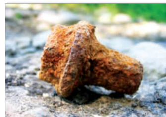
Fig. 6.3: Rust in iron
